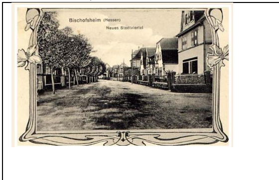
View of Mainzer Straße towards Gustavsburg ca. 1910.
