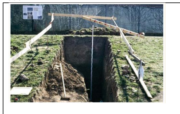
The approx. 2.7-metre-deep test pit at the embankment.
