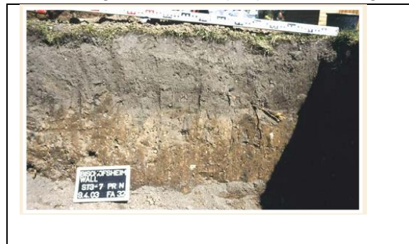
The dig made the stratification in the side of the embankment visible.
